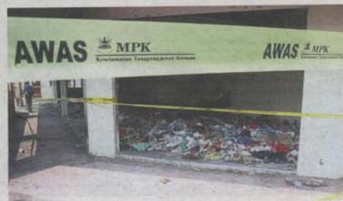
Rubbish has not been cleared from the shophouse along Jalan Jasmin 8.
